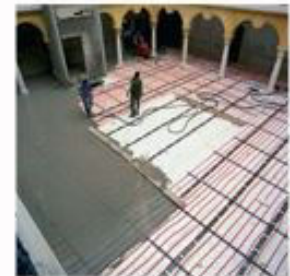
Step 4: Covering the pipes with Screed
