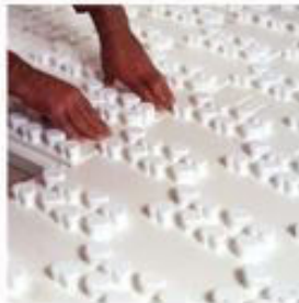
Step 2: Installation of the Insulated Board
