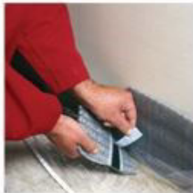
Step 1: Installation of the Edge Insulation Strip
